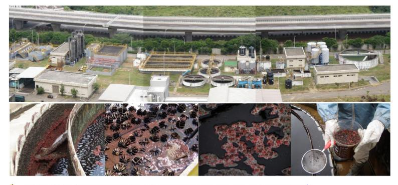
♣ Bali landfill leachate treatment plant: Flow rate: 800 CMD ,Nitrogen Loading: 480 kg-N/d
